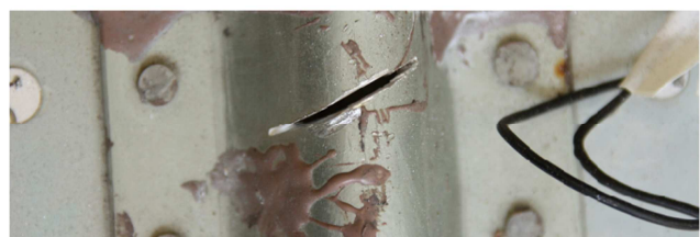
Fig. 3. Last stage of damage induced
